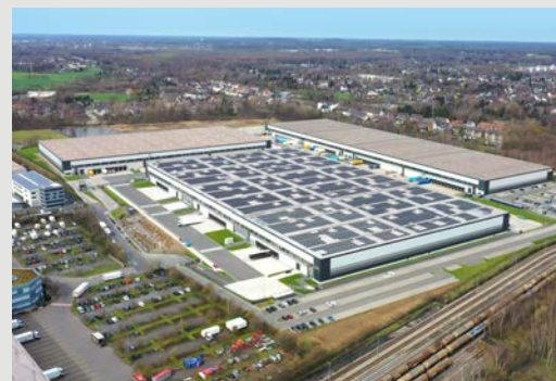
SEGRO Logistics Park Oberhausen
